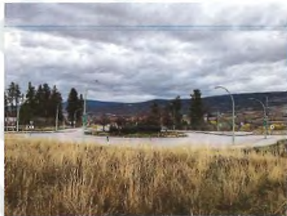
Photo 4. The roundabout at the north extent of the alignment
