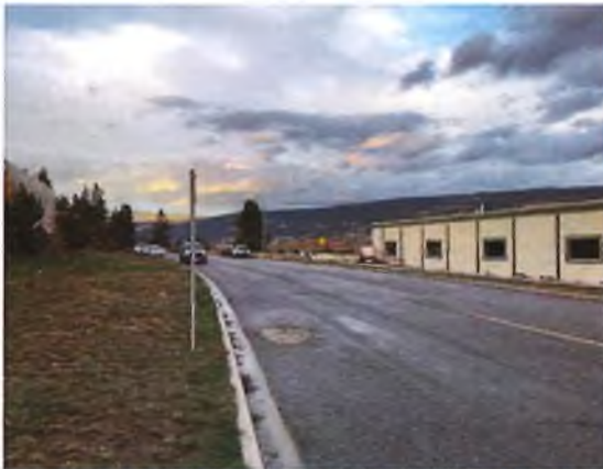
Photo 1. Conditions along existing Hollywood Road, viewing north
